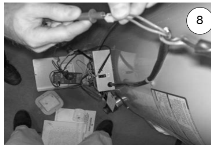
8 Checking continuity of upper sensor wire harness.
